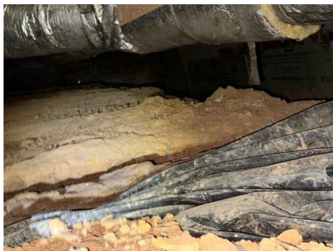
South Exposed Ground-Vapor Barrier Removed
