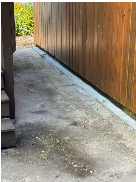
Recent Concrete Work-Southside
