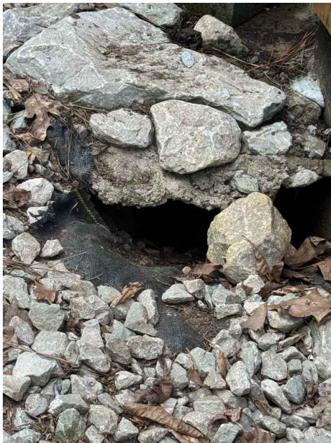
Erosion Hole-Southeast 2
