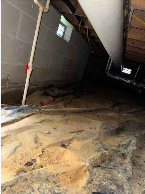
Crawlspace Entry West
