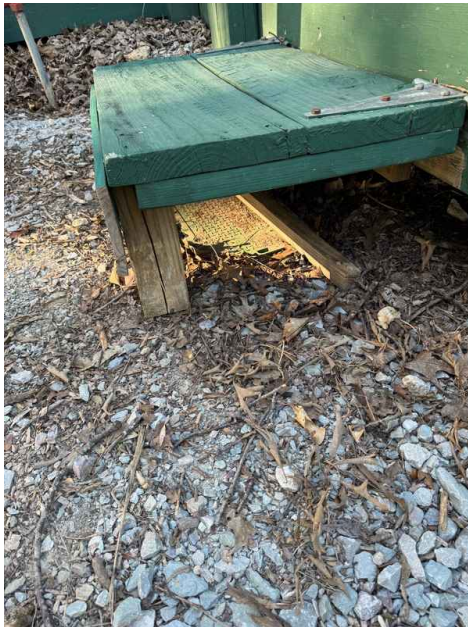
Shut-Off to Workshop 2
