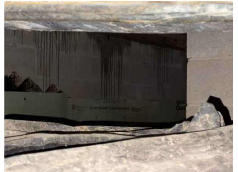
Basement Wall with ISO Board
