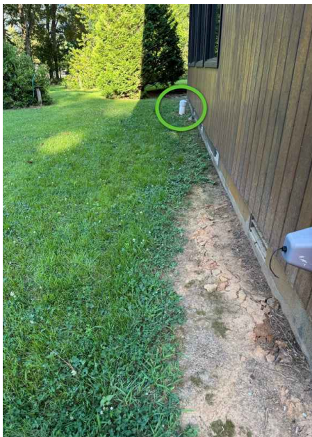
House Water Shut-Off
