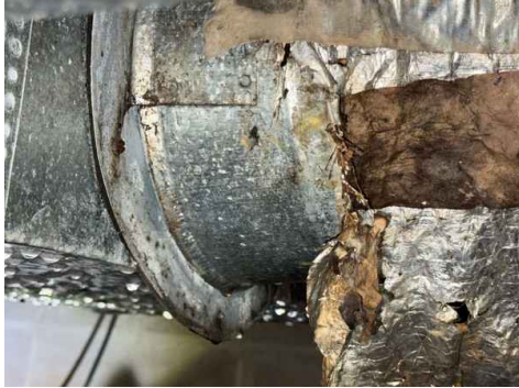
Missing Insulation
