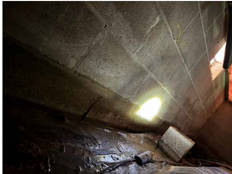
Crawlspace Middle Support Wall
