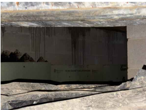
Basement Wall with ISO Board 2
